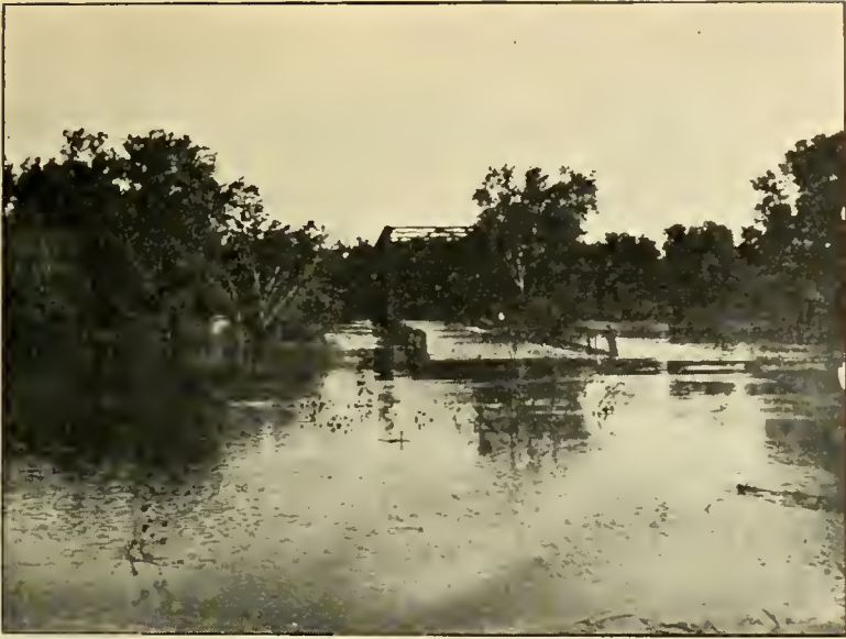
VIEW FROM SOUTH SIDE OF WEST BRIDGE OVER THE SOLOMON RIVER.
